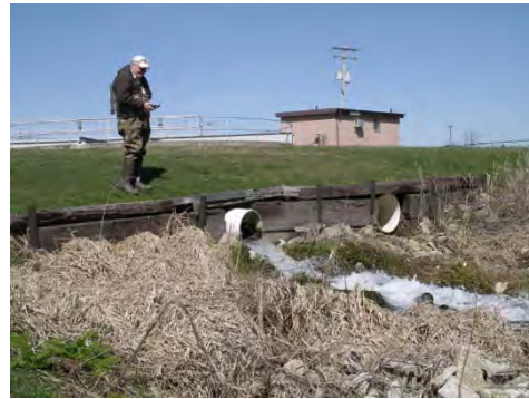
Abingdon Wastewater Outfall
