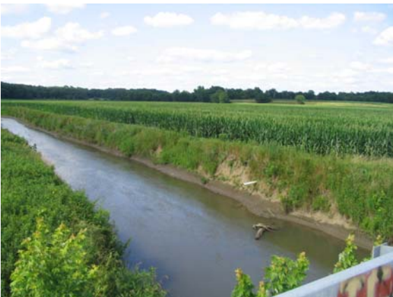
Mauvaise Terre Creek, along Willow Branch Rd
