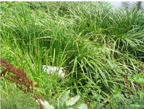
Culverts draining to Morgan Lake (adjacent to Mauvaise Terre Lake).
