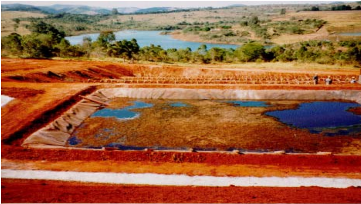
Figure 5-17. Sulfate-Reducing Bacteria Reactor
