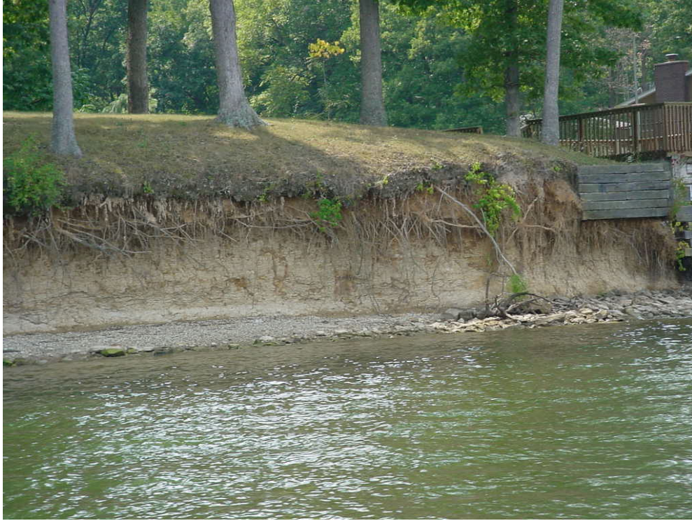
Lake Sara (Segment RCE). Severe bank erosion (IEPA photo)
