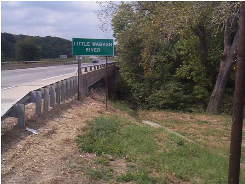
Little Wabash River Bridge
