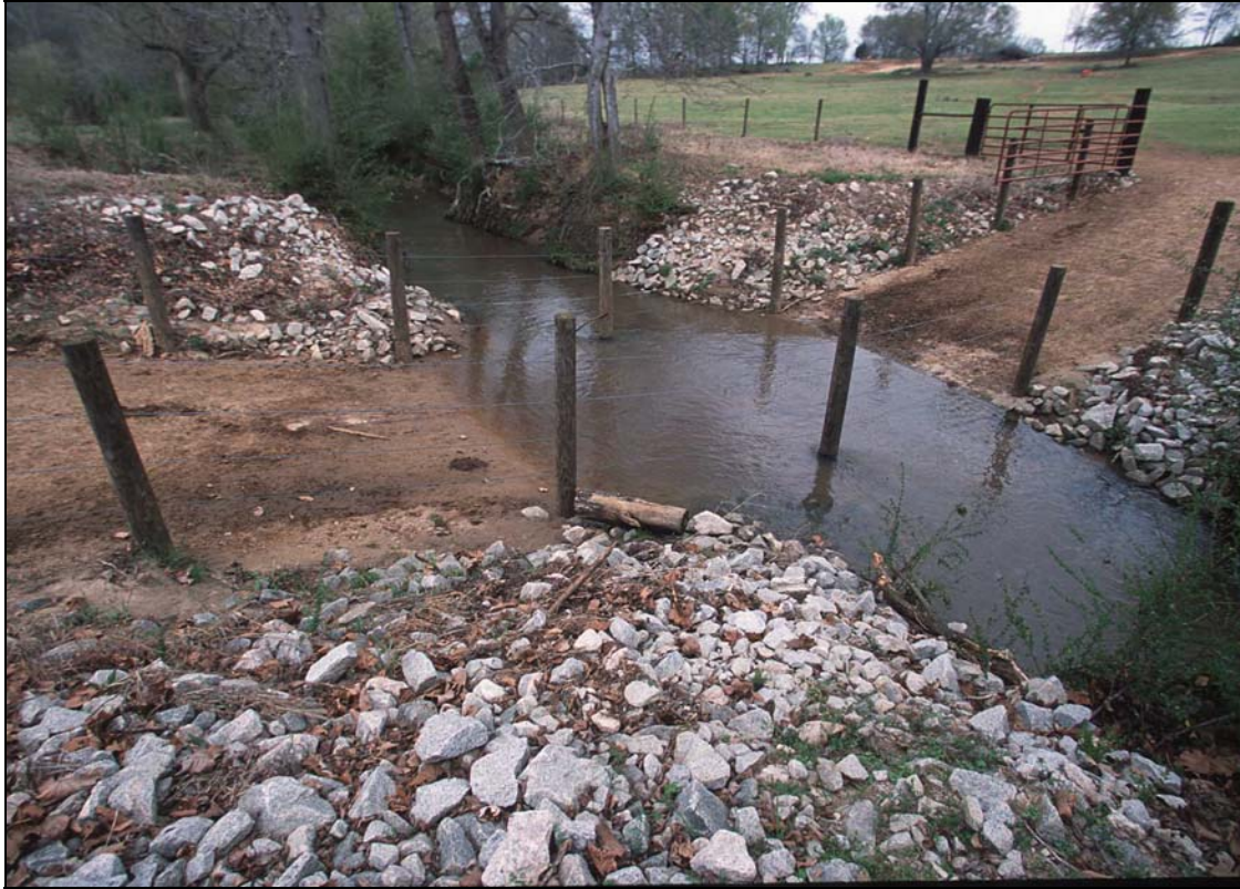
Figure 4-6. Restricted Cattle Access Point with Reinforced Banks.
