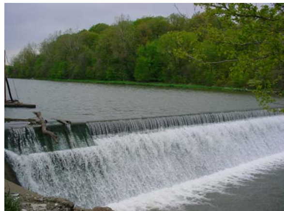
Figure 2-2. Georgetown Lake spillway.
