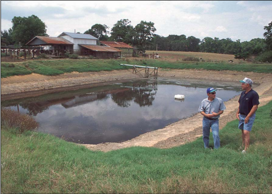
Figure 4-2. Waste Storage Lagoon.
