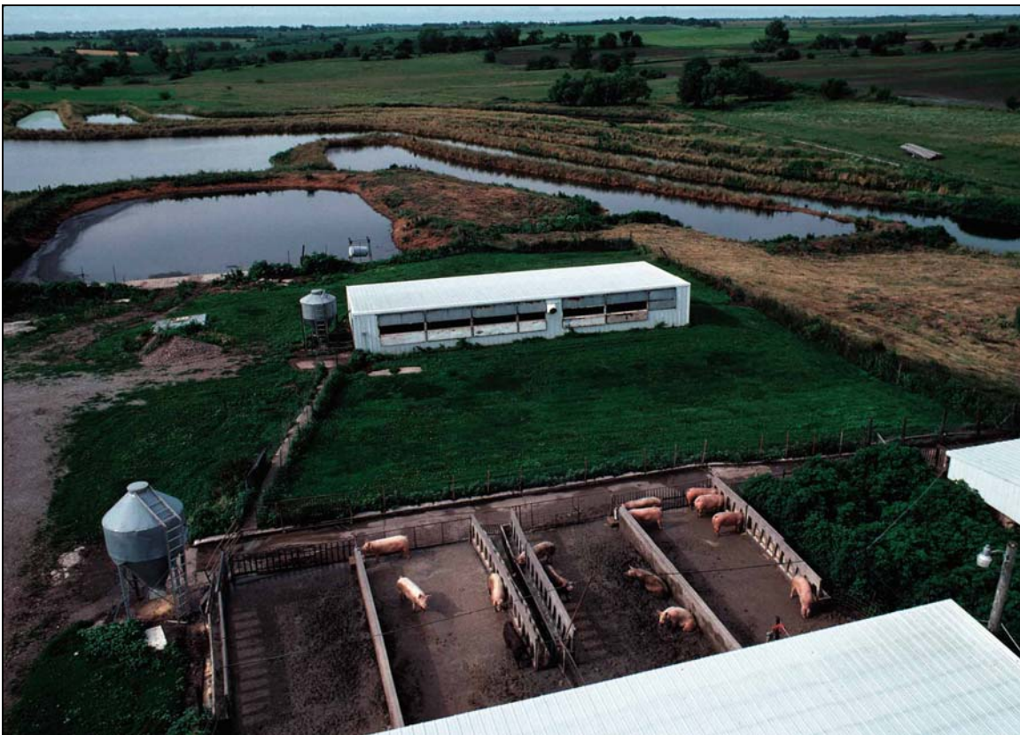
Figure 4-12. Constructed Wetland System for Animal Waste Treatment.
