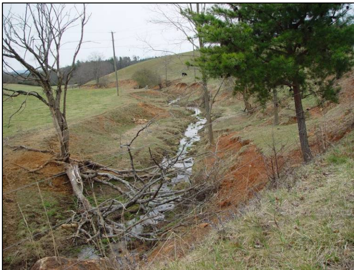
Figure 4-3. Typical Stream Bank Erosion in Pastures with Cattle Access to Stream.
