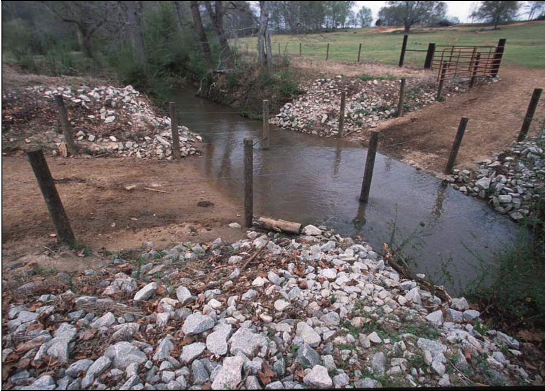
Figure 4-7. Restricted Cattle Access Point with Reinforced Banks.
