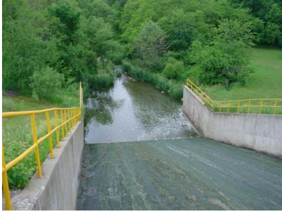
Spring Lake Dam 2 Discharging into Spring Creek
