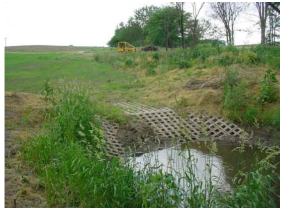
Block Chute on Lewis Farm in Farmers Fork (East Fork La Moine River Tributary) Watershed
