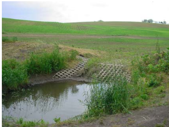
Block Chute on Lewis Farm in Farmers Fork (East Fork La Moine River Tributary) Watershed
