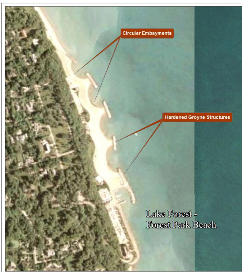
Figure 3-7. Example of Physical Structures at Shoreline Segments
