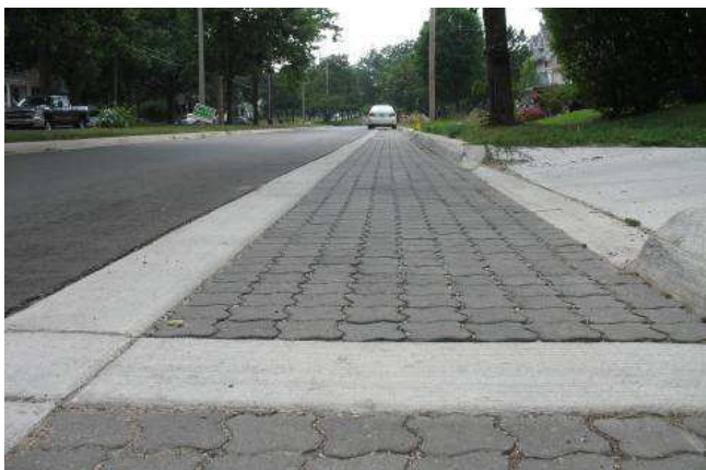
Figure 11. Porous pavement example.
