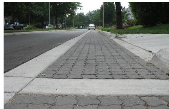
Figure 9. Green infrastructure examples: top - residential rain garden; bottom - permeable pavement.
