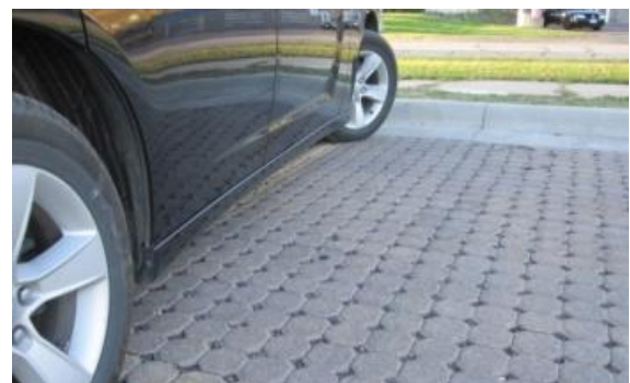
Figure 23. Green infrastructure examples: top - bioswale in parking lot; middle - green roof; bottom - permeable pavement.
