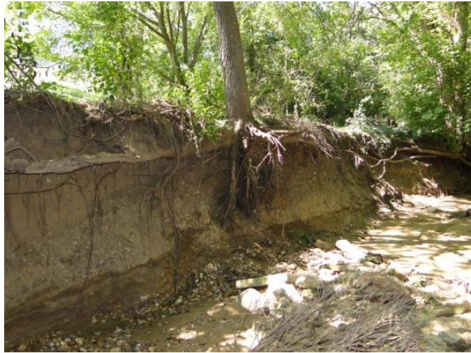
Figure 6. Eroding bank within North Farm Creek subwatershed.
