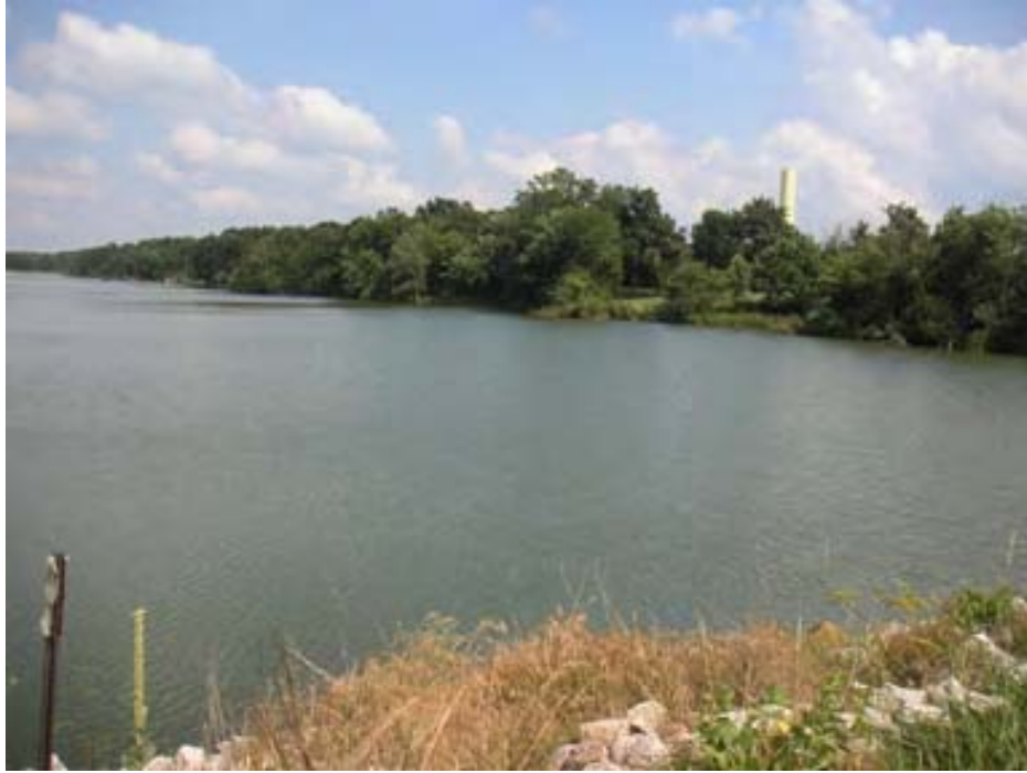
Palmyra-Modesto Lake from road between golf course lake and Terry Park lake (tower is water treatment plant)
