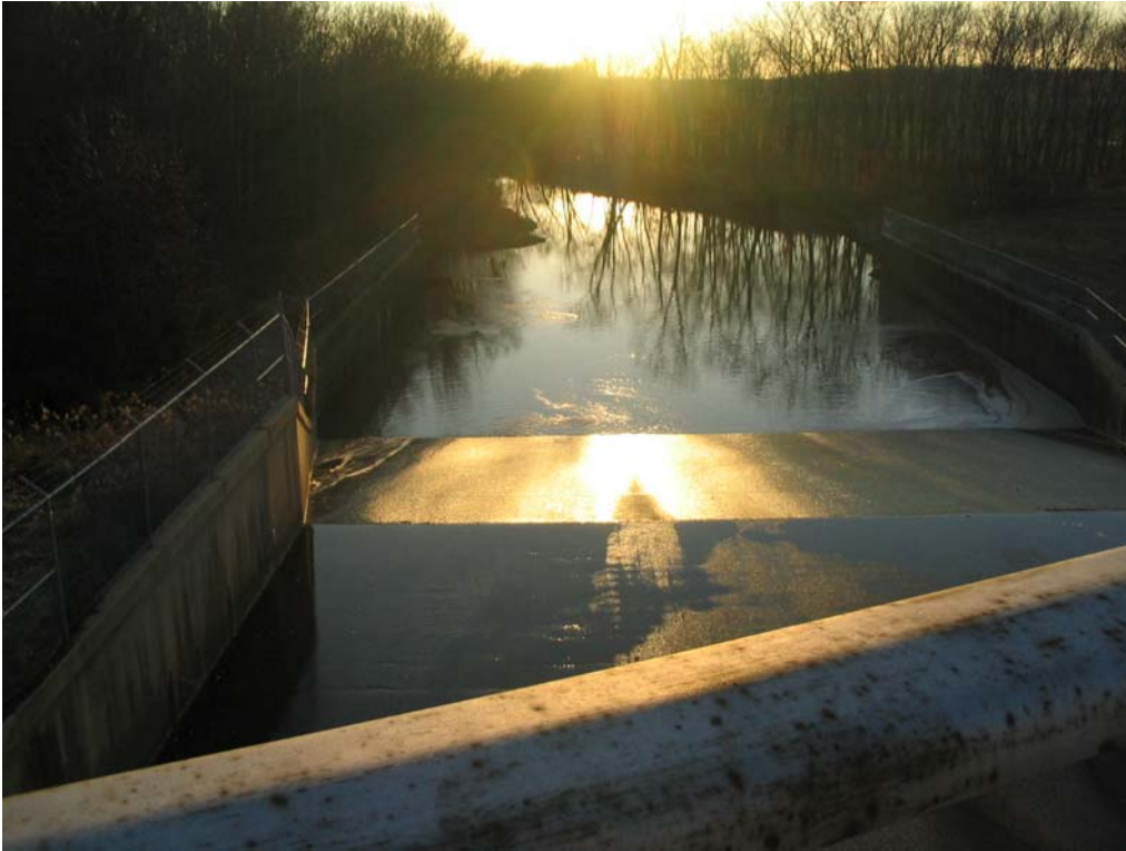
Looking downstream of dam at Highland Silver Lake outlet
