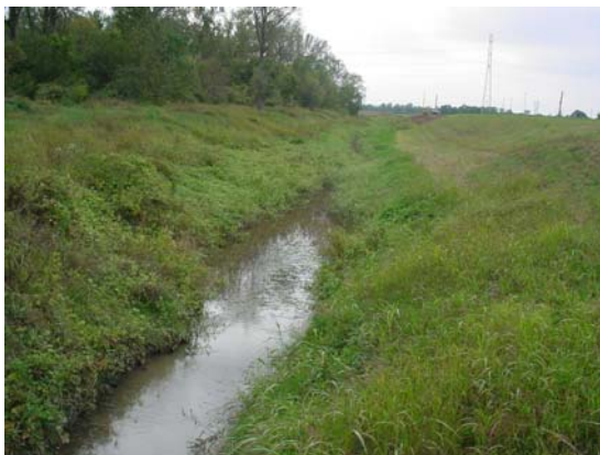
Cahokia Canal at Route 162 Looking South
