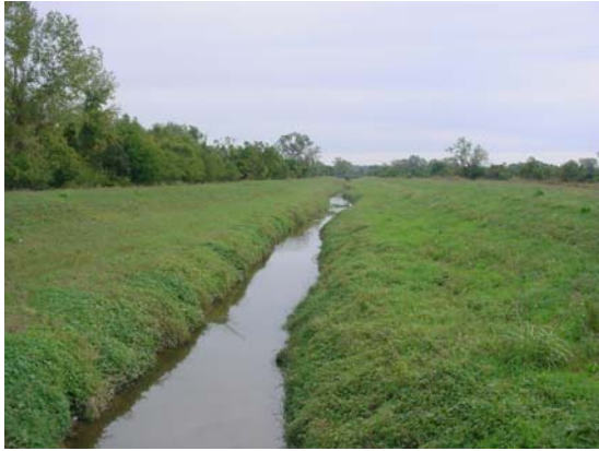
Canteen Creek at Sand Prairie Road Looking East
