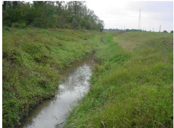
Cahokia Canal at Route 162 Looking South
