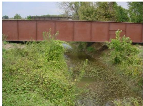
Cahokia Canal at Route 162 Looking North
