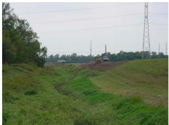
Cahokia Canal at Route 162 Looking South (Construction Activity)
