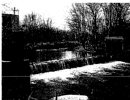
The movable South Fork Dam can be raised to back water into Horse Creek (center) for pumping into Lake Springfield when the water level drops in the lake.
