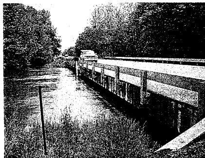
Lake water level is determined by flow from its feeder creeks. In Lick Creek shown here, spring storms bring the stream to flood stage (above), whereas it can dry up into a series of disconnected pools in summer (below).
