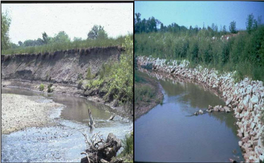
Figure 44 - Rip-Rap Stabilization
