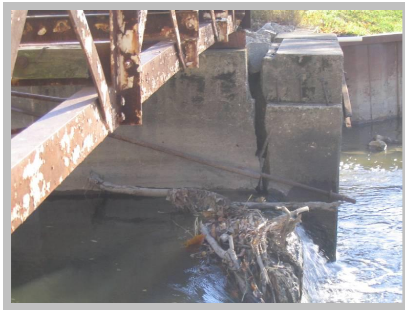
Figure 2- 3 - Left abutment, significant crack
