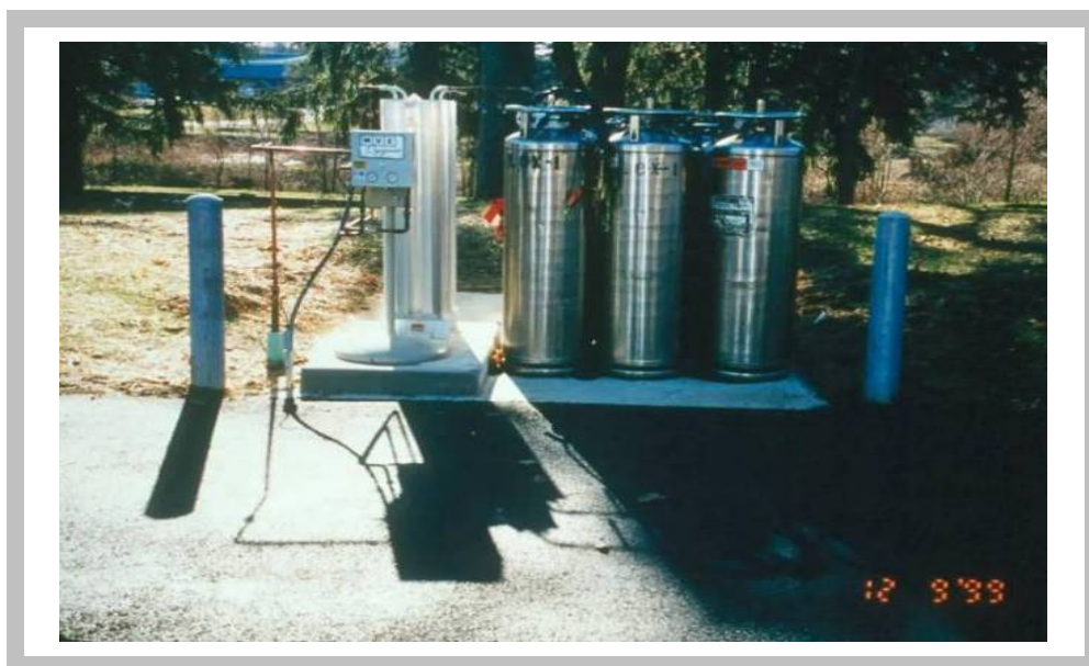
Figure 6-3 - Low Head Oxygenators with liquid oxygen cylinders
