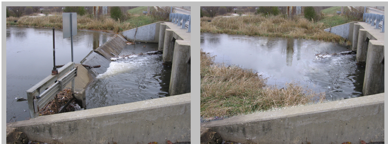
Figure 7-4 - Churchill Woods Outlet Before and After Dam Removal
