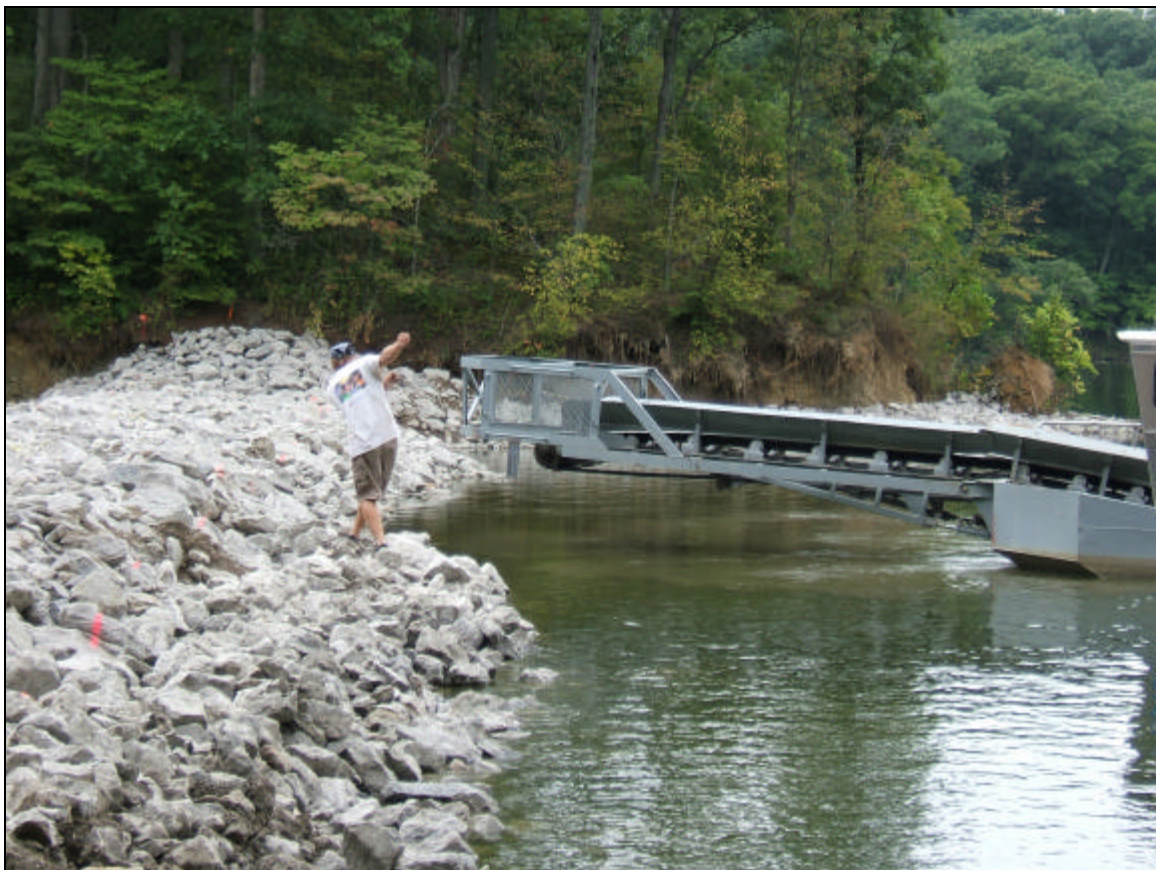
Figure 7. Barge building dam, shoreline work in background
