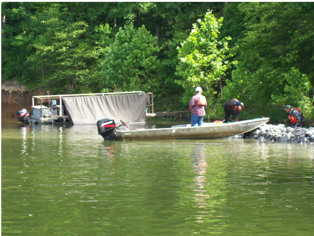
CREW PLACING FILTER FABRIC IN ADVANCE OF RIPRAP PLACEMENT
