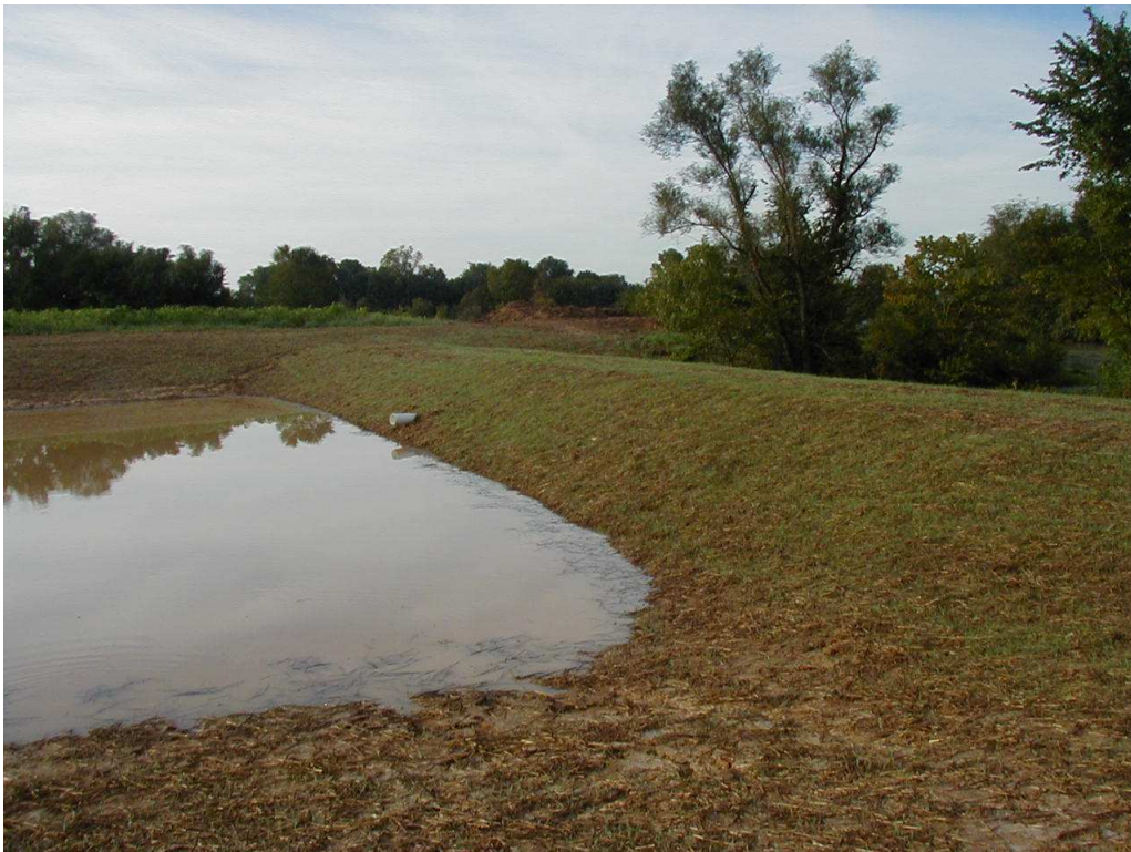
SEDIMENT / NUTRIENT DETENTION BASIN #2: UPSTREAM SLOPE OF DAM
