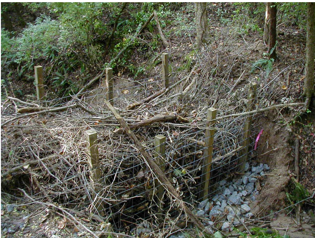
GULLY STABILIZATION – STRUCTURE TYPE 2
