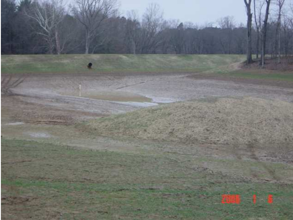
SEDIMENT / NUTRIENT DETENTION BASIN #1: BASIN AND UPSTREAM FACE OF DAM PRIOR TO FILLING
