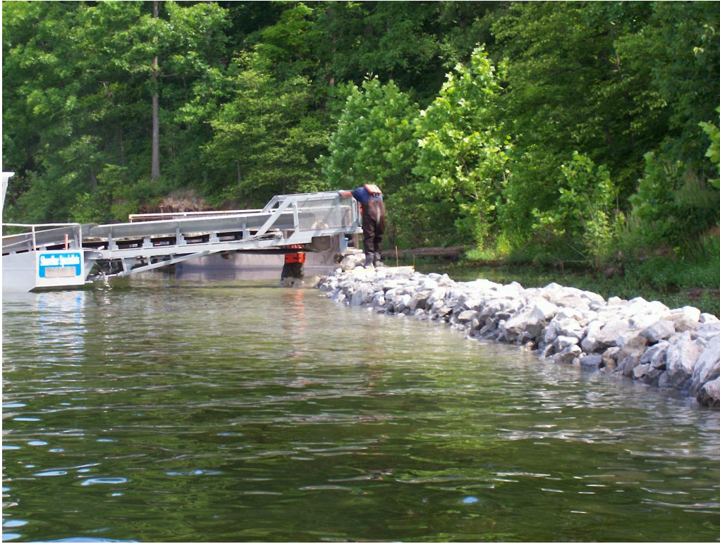
RIPRAP PLACEMENT ON INSTALLED FILTER FABRIC
