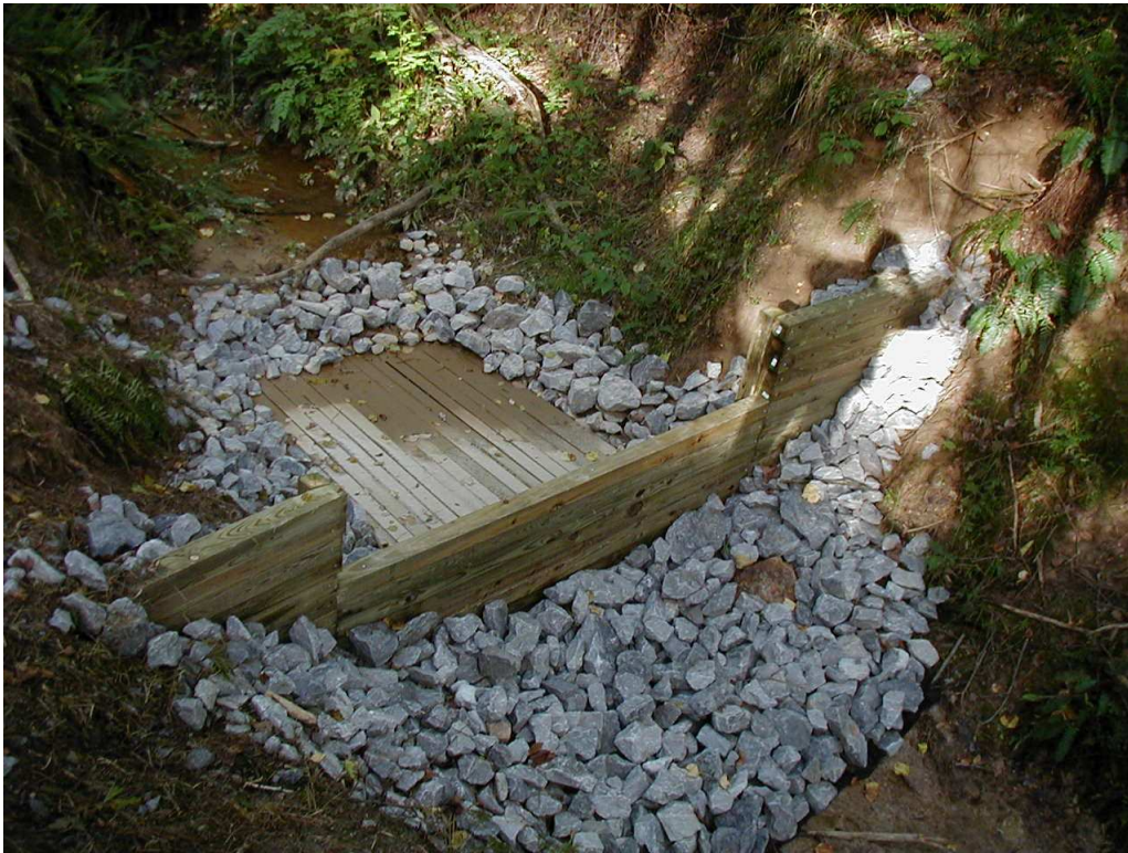
GULLY STABILIZATION – STRUCTURE TYPE 3
