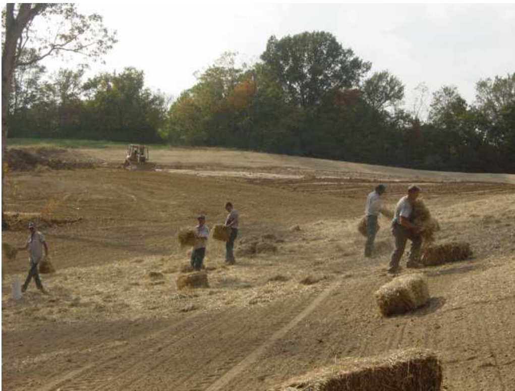
SEDIMENT / NUTRIENT DETENTION BASIN #1: STRAW MULCH APPLICATION
