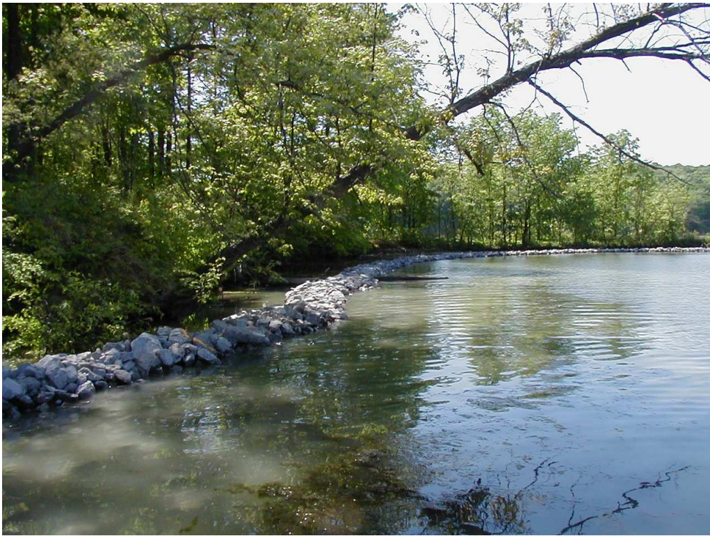
FINISHED PRODUCT: OFFSHORE BREAKWATER USING RR 4 RIPRAP
