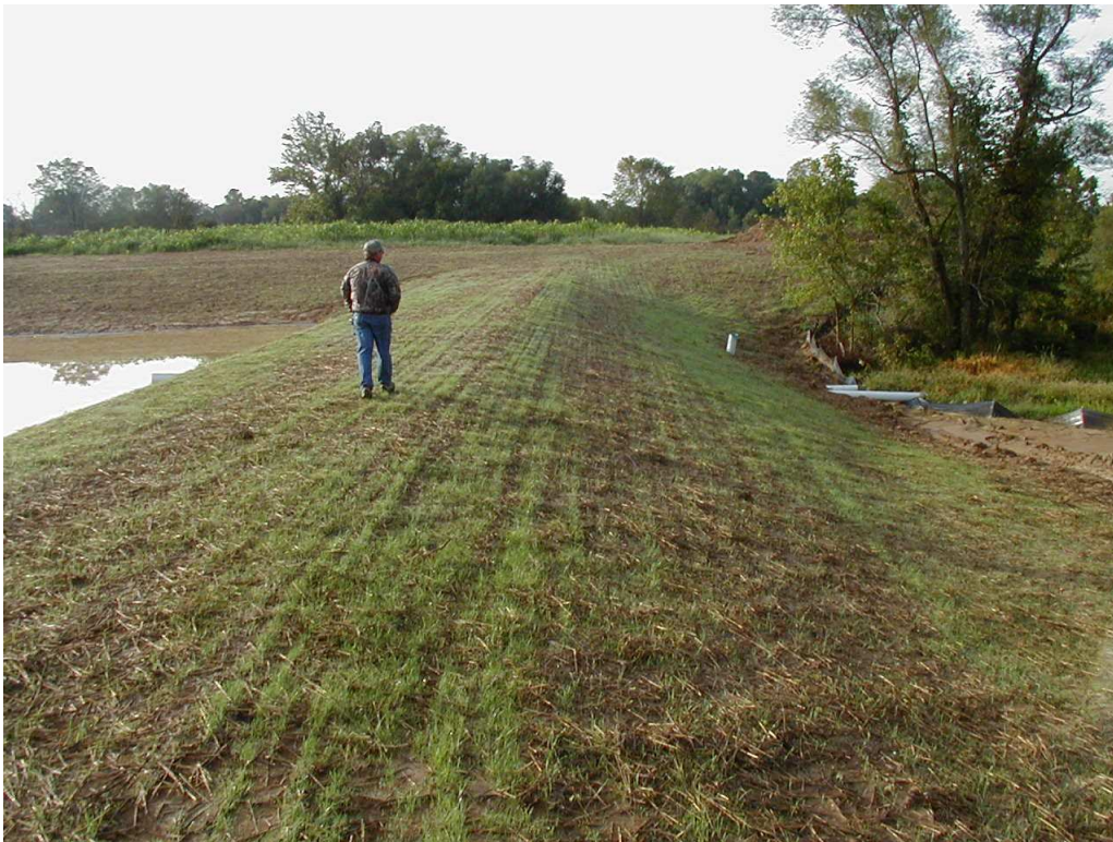
SEDIMENT / NUTRIENT DETENTION BASIN #2: DOWNSTREAM SLOPE OF DAM
