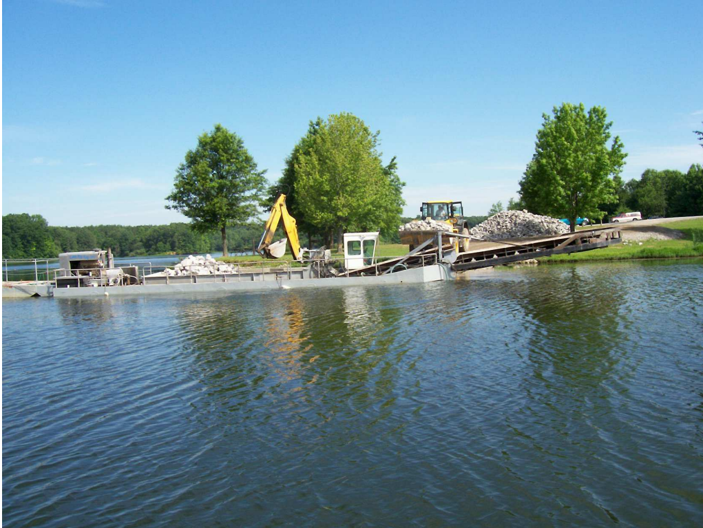
ENDLOADER LOADING RR 4 RIPRAP ON MECHANICAL BOAT
