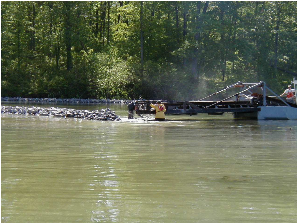
RIPRAP PLACEMENT USING MECHANICAL BOAT
