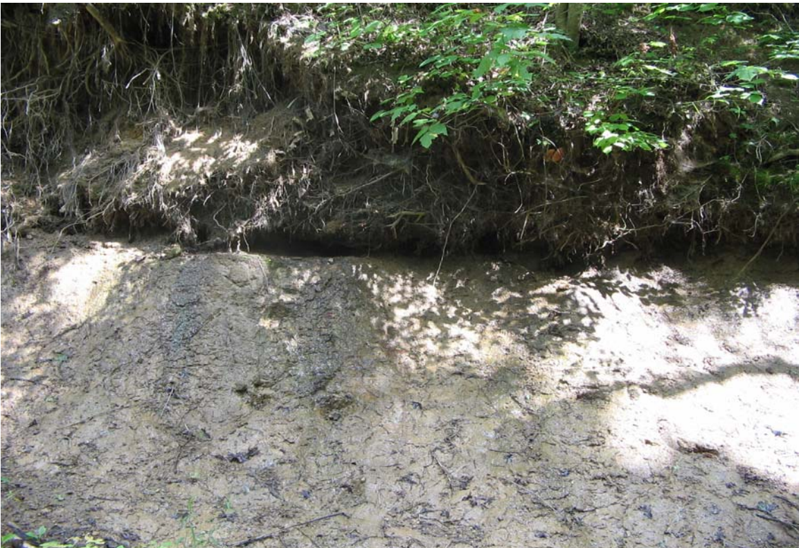
Fig. 33 Geotech problem at interface of silt over glacial till at Cross Section 2
