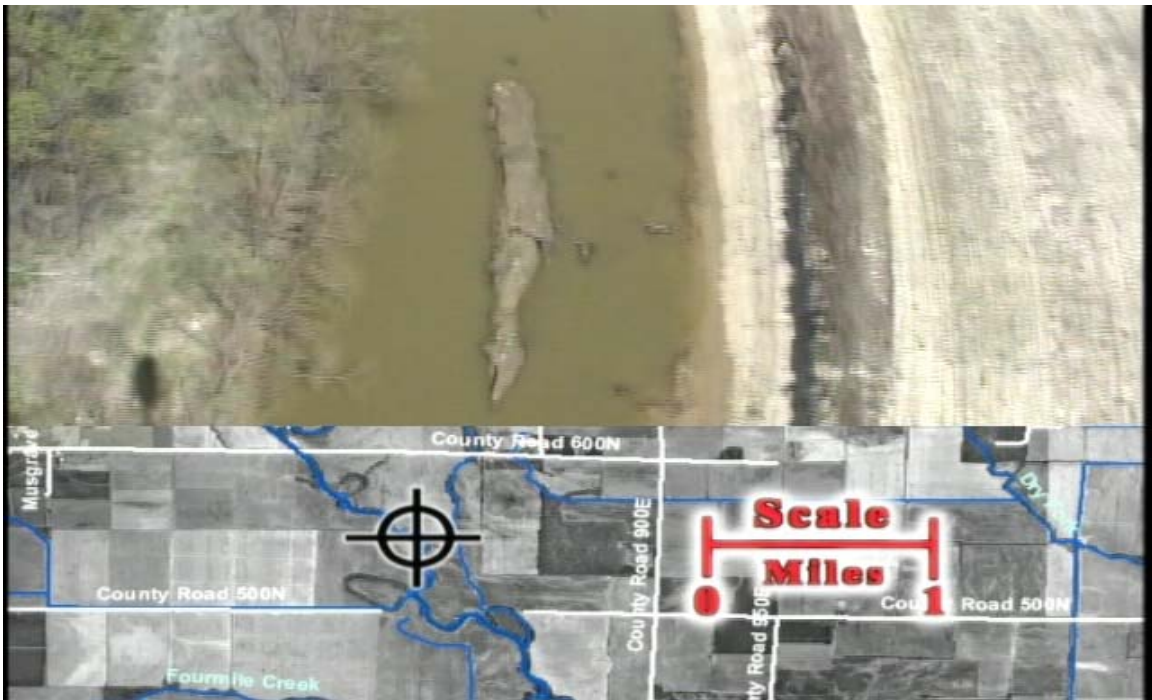
Fig. 26 Eroding bend at DVD 46:10. What appears to be a central bar of deposition is really a pedestal of residual material about 2 to 3 feet above the current channel bed.
