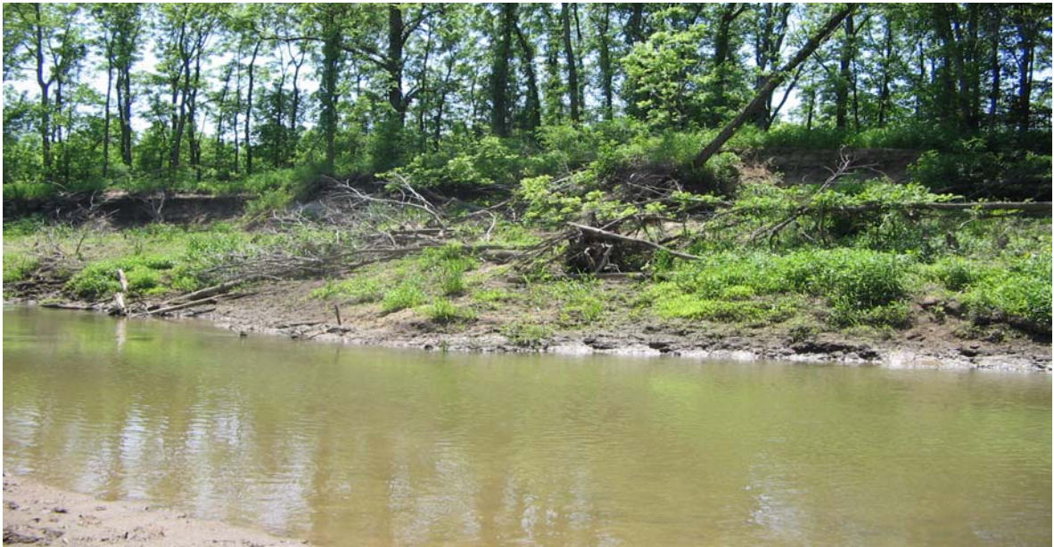
Fig. 4 Geotech Failure near X-sec 6 below Interstate 57.
