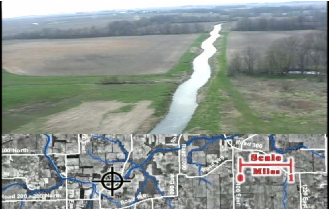
Fig. 11 Channelized reach with no woody riparian area; notice meanders forming in channel that will tend to undercut stable banks.
