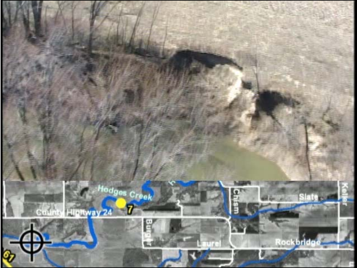
Geotechnical failure just above the confluence of Hodges and Macoupin Creek
