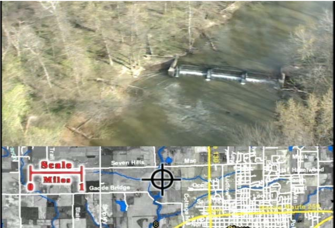
Figure 12 Structure below water treatment plant at Olney—7:35 DVD tape 2
