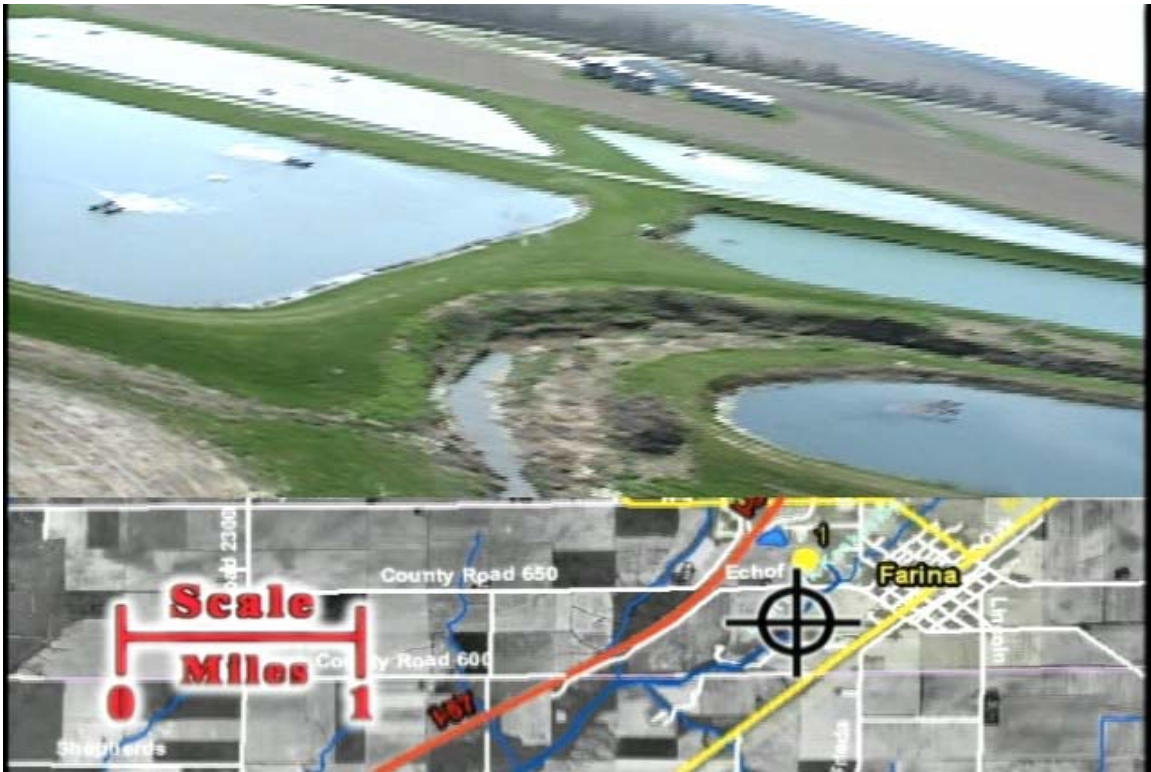
East Fork Kaskaskia erosion site between Farina Sewage Treatment Lagoons
