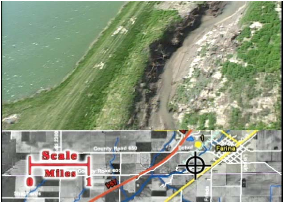
East Fork Kaskaskia eroding into embankment of Farina Sewage Treatment Lagoon
