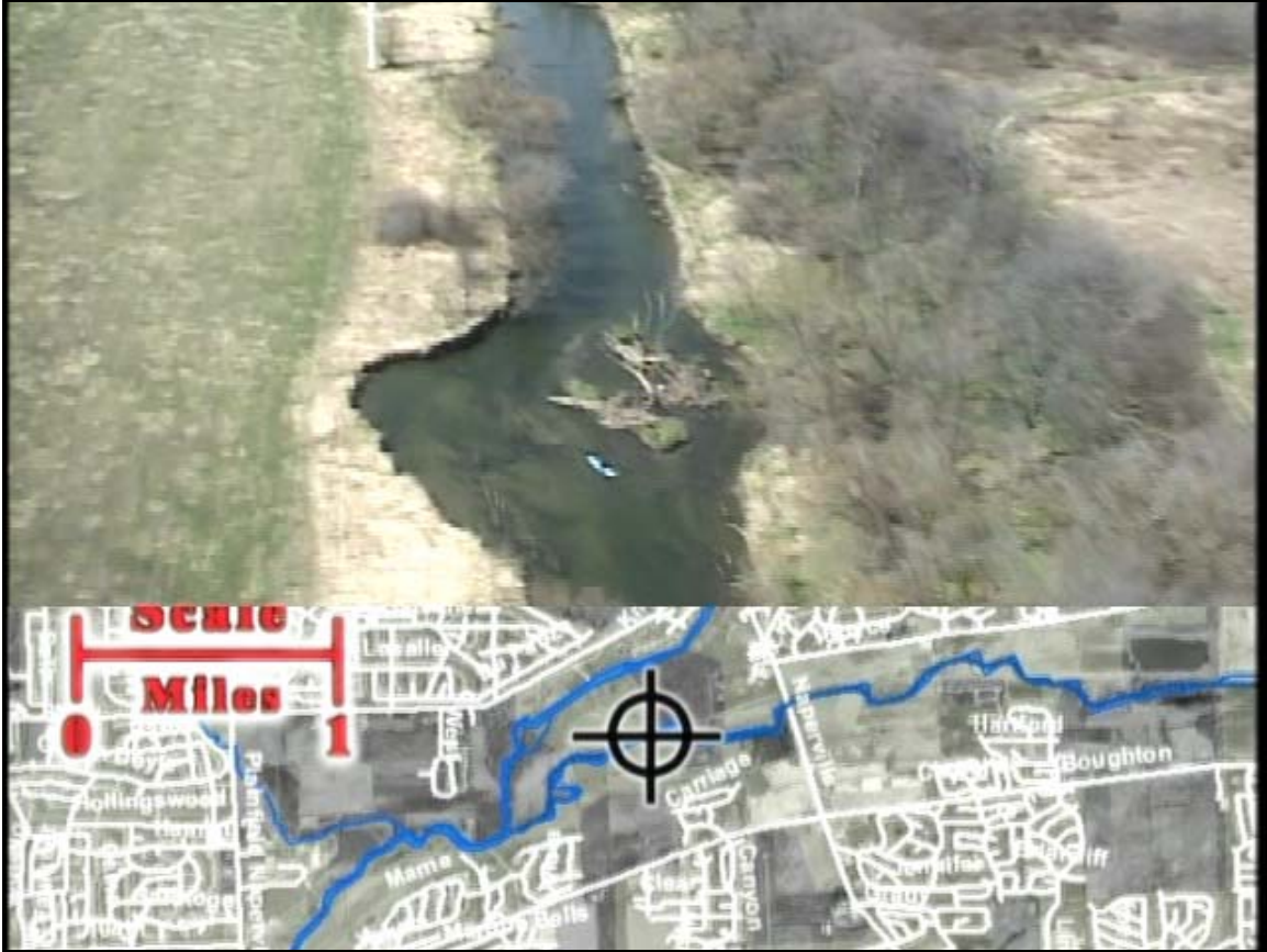
Fig. 18 Logjam, lateral bank erosion and sediment deposition in Chapter 4
