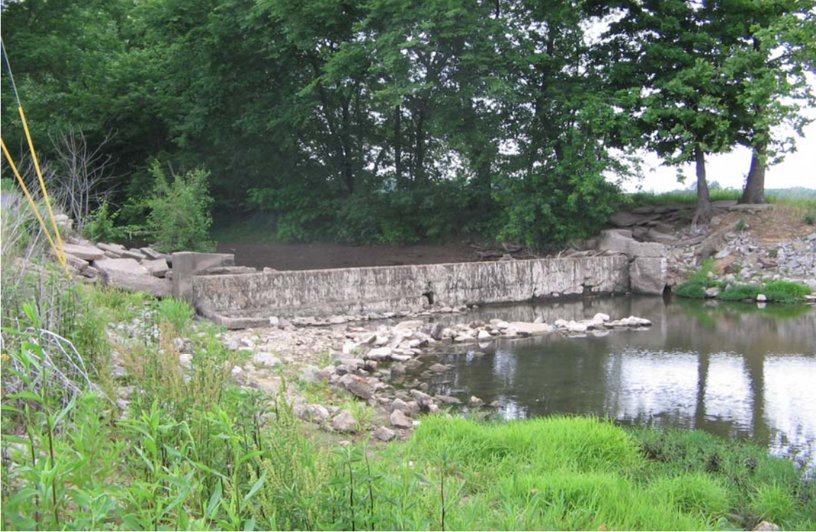
Fig. 4 Dam above Tolle Road. Only true grade control identified in assessment.
