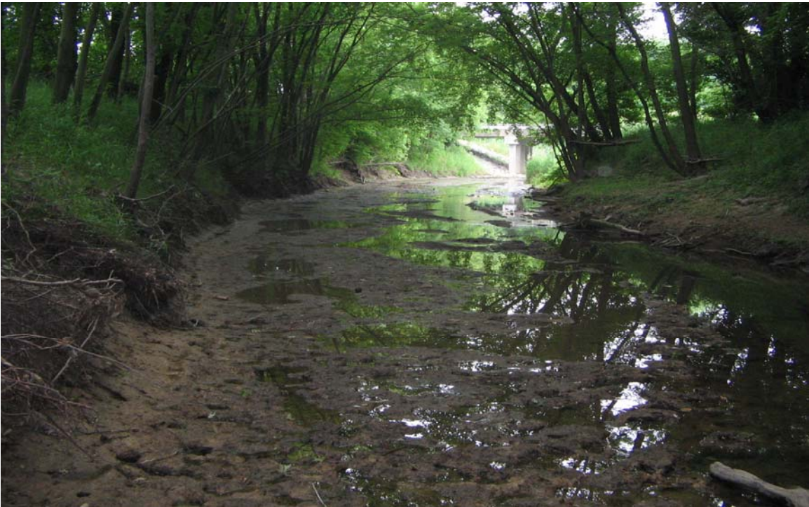
Fig. 7 Knickpoint above Road 1250N; bed is actively downcutting
