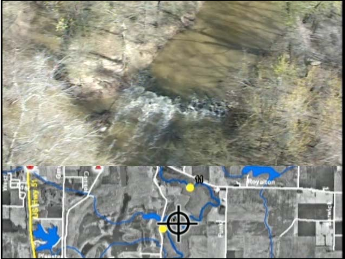
Fig. 19 Grade Control on DVD 2 at 11:20. Provides some re-aeration of flow.
