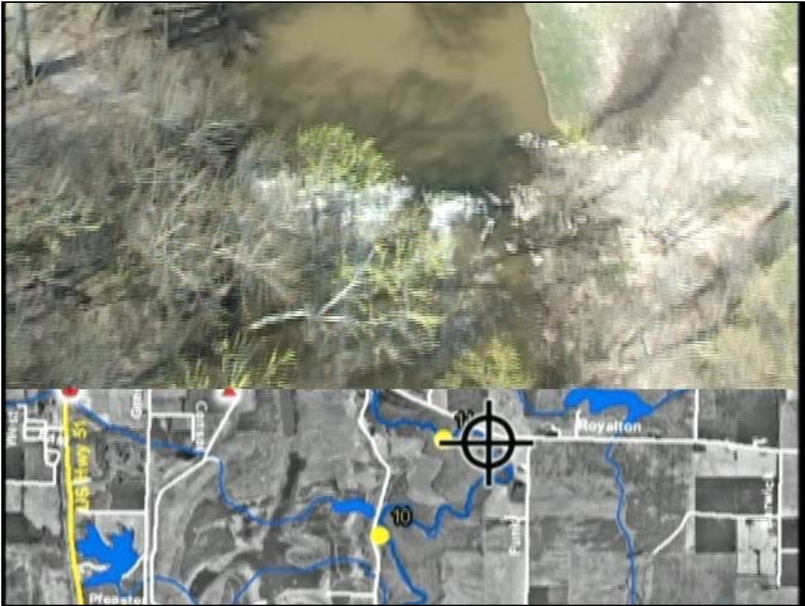
Fig. 18 Low water crossing on DVD 2 at 14:48 acting as grade control and providing some re-aeration.
