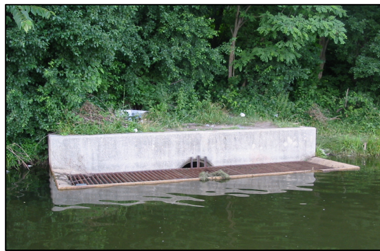
At this outlet structure, there was no flow out of the lake. The water level was measured with a ruler to be about 1 1/4 inch below the top edge of the spillway. The volunteer monitor thus recorded that the Lake Level was "Below normal by 1 1/4 inch."
