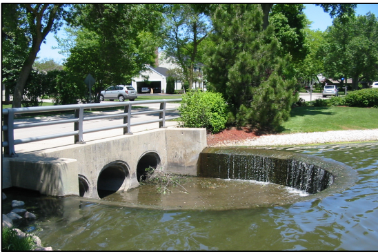
At this lake outfall structure, the water depth over the top, outer edge of the spillway was about 1/2 inch (measured with a ruler). The volunteer monitor thus recorded on the Secchi Monitoring Form that the Lake Level was "Above normal by 1/2 inch."
