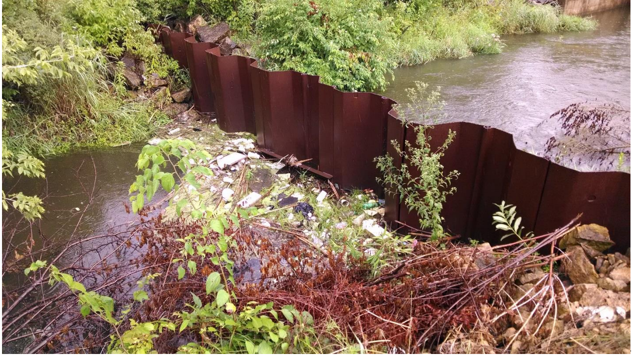
Figure 29 Kress Road sheet pile dam
