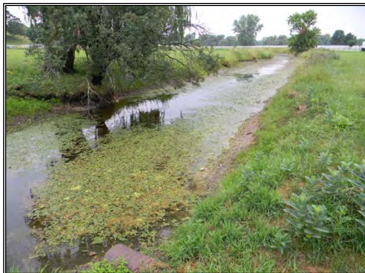
Channelization along Spring Creek; Reach 10 (SPCR10)
