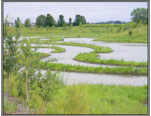
Properly designed/planted wet bottom naturalized detention at Arboretum Shopping Center
