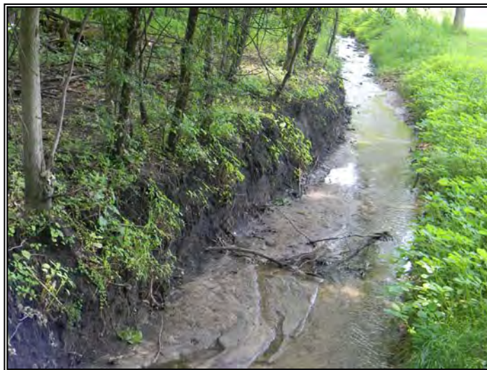
Highly eroded banks along Tributary H; Reach 2 (TRH2)
