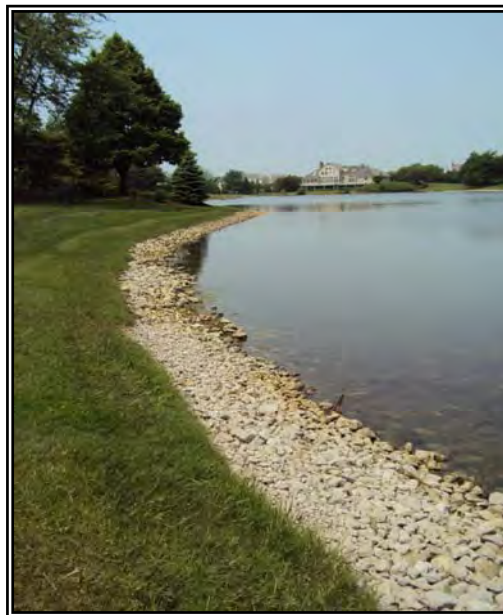
Typical older wet bottom detention found in the east portion of the watershed
