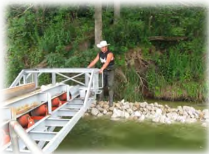
Application of Rock; Shoreline Stabilization
