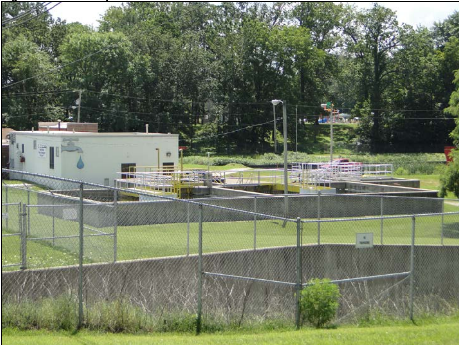
Figure 5. Salem City Water Treatment Plant
