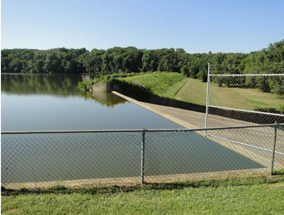
Figure 8. Lake Carlerville Spillway
