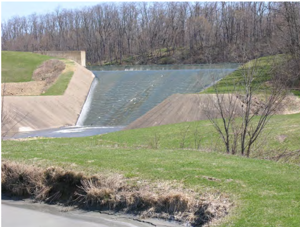
Figure 5-4. Canton Lake Spillway (base station RDD-T1)
