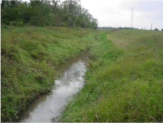
Cahokia Canal at Route 162 Looking South
