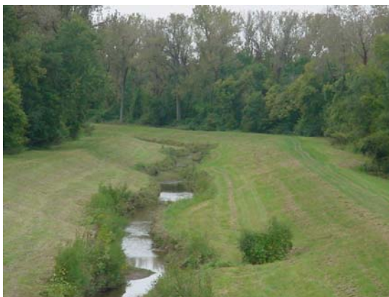
Harding Ditch Southwest of Lake Boulevard Looking North
