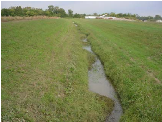
Harding Ditch at Bunkham Road Looking North
