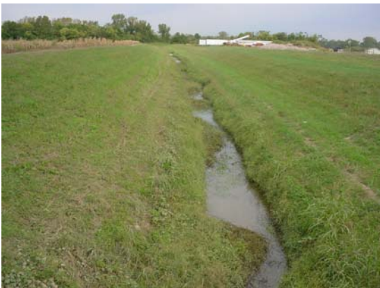
Harding Ditch at Bunkham Road Looking North
