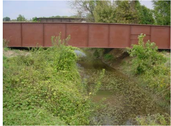
Cahokia Canal at Route 162 Looking North
