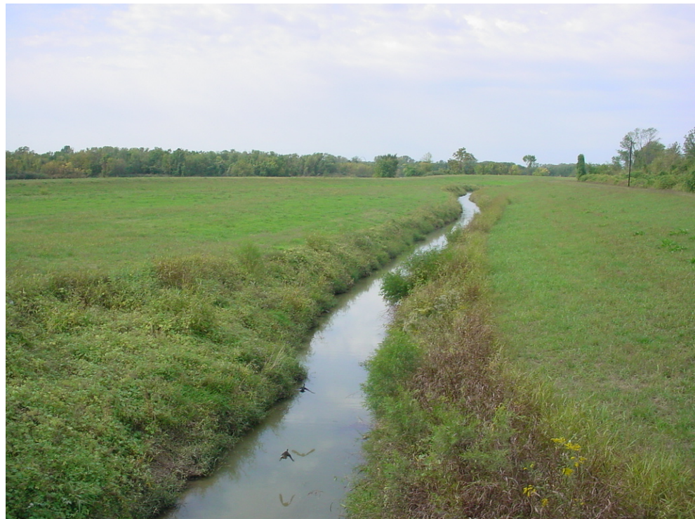
Cahokia Canal at Prairie Road
