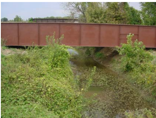
Cahokia Canal at Route 162 Looking North
