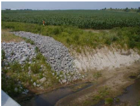
Walkers Creek looking northeast from the bridge at Illinois Routes 13/127.
