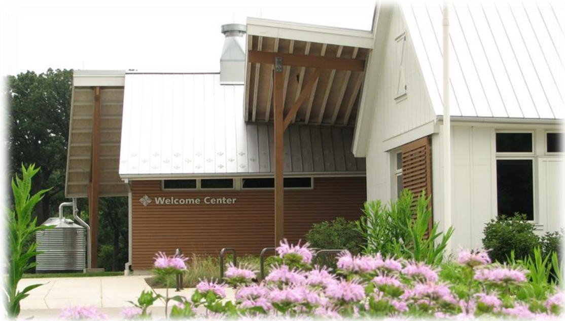
1 2 Figure 12: Ryerson Woods Welcome Center 56
