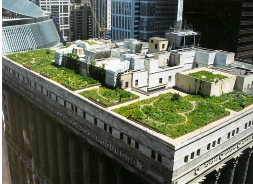
Figure 6: Chicago City Hall Green Roof
