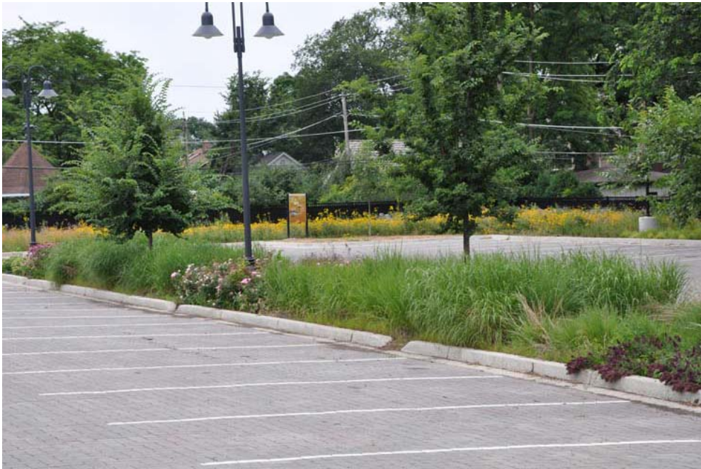
10 Figure 12: Elmhurst College West Hall Permeable Paver Parking Lot and Bioswales 65
