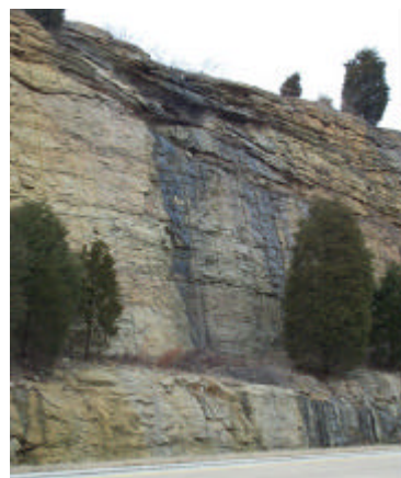
Groundwater seeping out at a road cut in Southern Illinois off Interstate 24.
