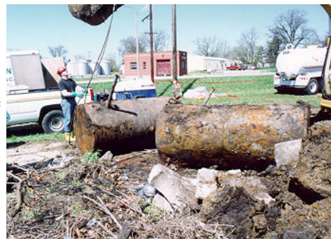
Removal of leaking underground storage tanks.
