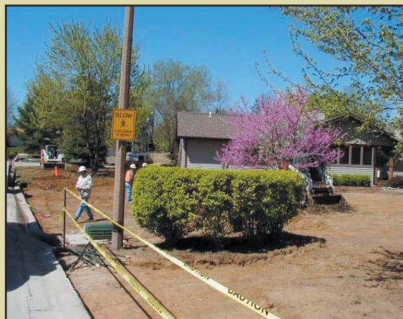
After removal of contaminated soil, clean fill soil is brought in, to be followed with topsoil and sod application in this yard, near the former St. Louis Smelting and Refining facility.
