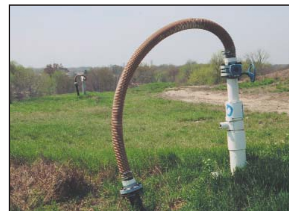
Methane gas controls at landfill
