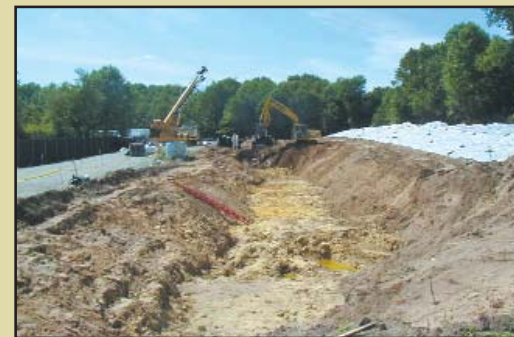
Removal of chemical waste disposal trench
