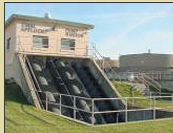
Mechanical screws carry finished effluent from a wastewater treatment plant up an incline for discharge into a nearby receiving stream.
