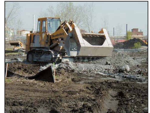
Grading and filling at the Chicago Manufacturing Campus
