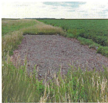
Denitrifying Bioreactor in Piatt County.
