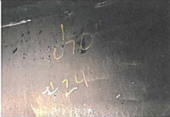
Description: Arc gouged area under tray ring 24. .070 x 1"
